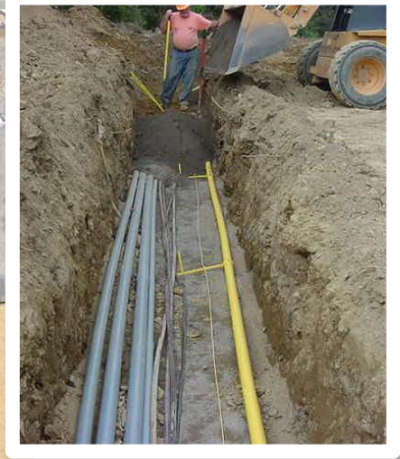
Joint trench under brick banding
